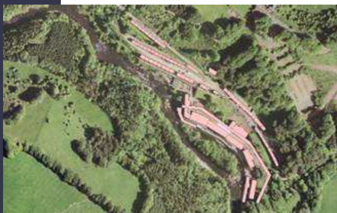
©Crown copyright, RCAHMS
